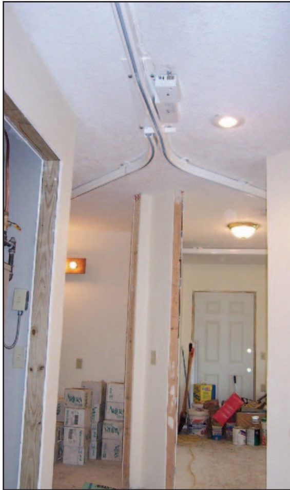
The extruded aluminum ceiling track guides Lisa's lift, transferring her easily throughout her new home.
