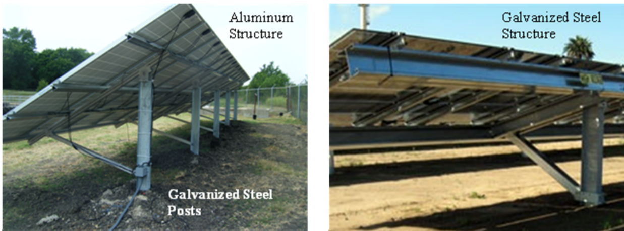
Figure 1: Utility Scale Ground Mount Systems
