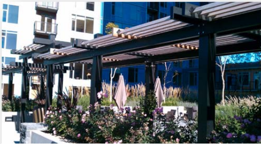
Illustration 1: Custom designed extruded aluminum railing system, aluminum trellis and barbeque canopy, Hydro Architectural Products.
